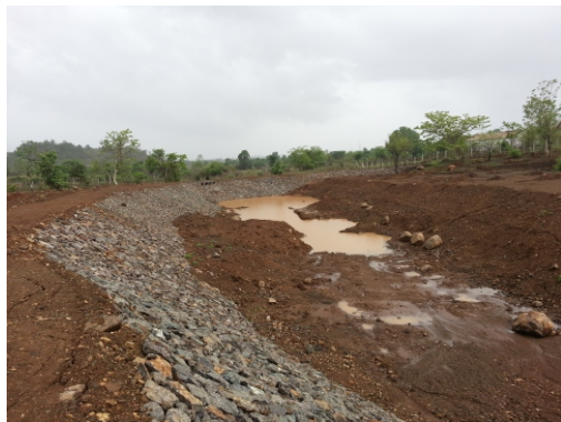
Lake excavated over 1.5 acres and rain water collected. Soil being very fine, pond liner was not used. Stages of the lake over 3 years are shown in the pictures.
