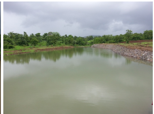
Lake excavated over 1.5 acres and rain water collected. Soil being very fine, pond liner was not used. Stages of the lake over 3 years are shown in the pictures.
