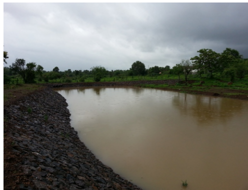
Lake excavated over 1.5 acres and rain water collected. Soil being very fine, pond liner was not used. Stages of the lake over 3 years are shown in the pictures.
